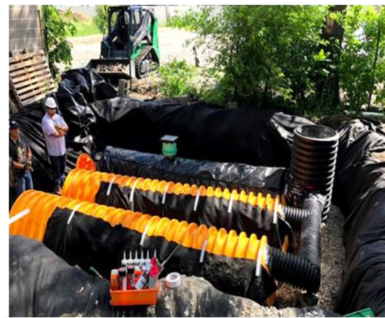
Below Ground Cistern
