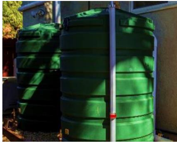
Above Ground Cistern
