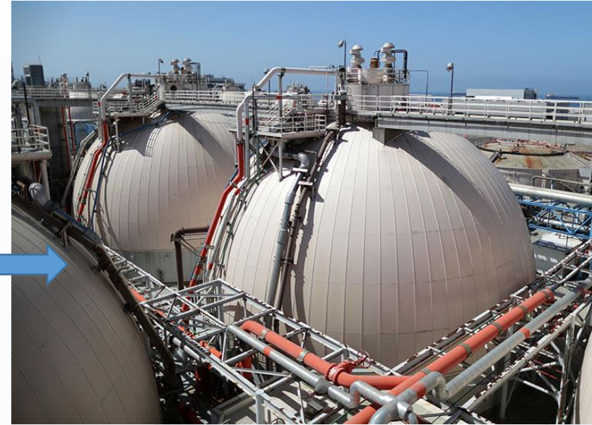
Hyperion Treatment Plant
