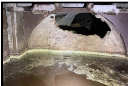
Existing Concrete Plug
