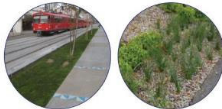
Vegetated Filter Strip typ max slope = 6-33%
