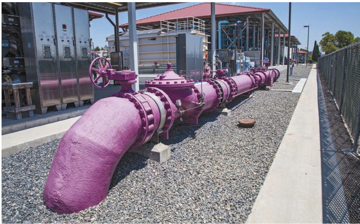
Above, the Leo J. Vander Lans (LVL) facility, located in Long Beach, treats recycled water used for injection wells at the Los Alamitos Barrier to prevent seawater intrusion. Left, a purple pipe at LVL carrying treated water from the Los Angeles County Sanitation Districts' Long Beach Water Reclamation Plant; water undergoes three more treatment processes at the facility.
