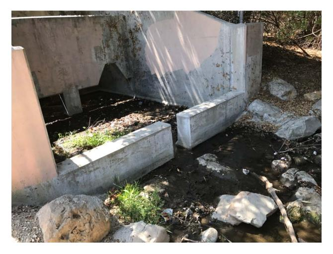
**Photo 11 -** This shows the water culvert and where the excess water from the hillside finally is captured. It empties out into the small stream that runs past the collection of oak trees in Area 2.
