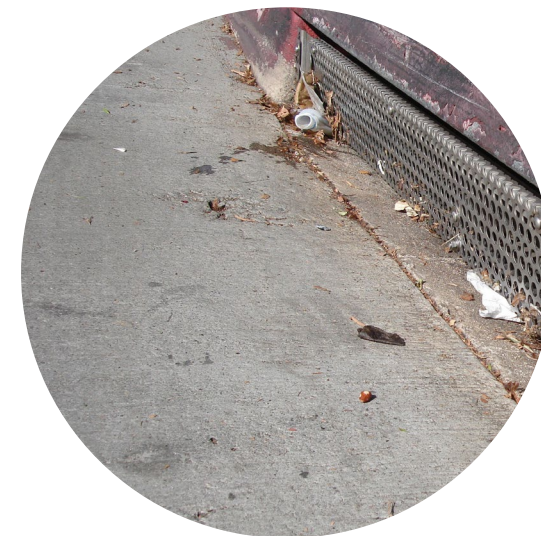
Trash capture devices installed
