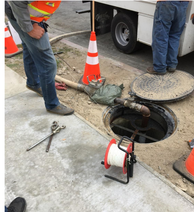
City of LA (North Hollywood) full-scale drywell test
