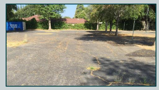
DETERIORATED ASPHALT PAVEMENT (BEFORE)
