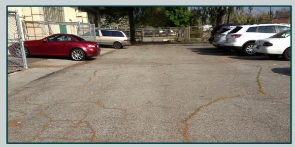
**DETERIORATED AC PAVEMENT (BEFORE)**
