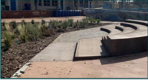
BIORETENTION AND PERVIOUS PAVERS BY AMPHITHEATER
