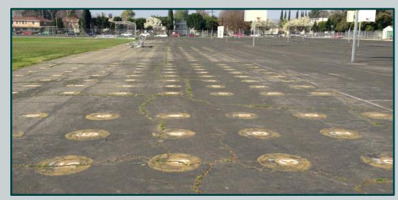
DETERIORATED ASPHALT AT PE YARD (BEFORE)
