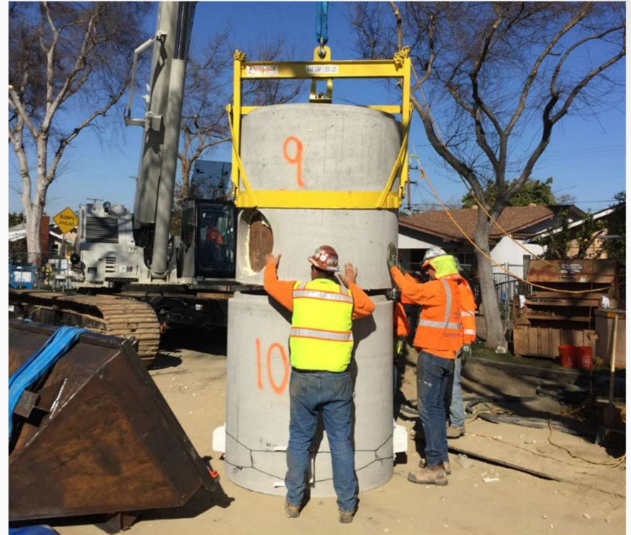
Example photos of drywell installation
