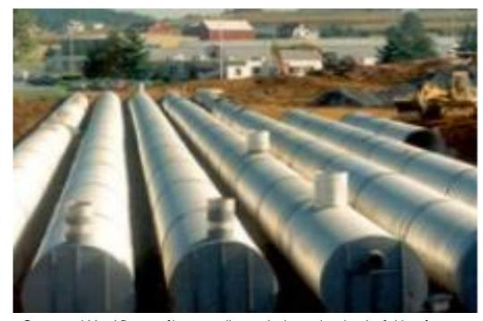
Corrugated Metal Pipe – infiltration galleys to be located under the field turf
